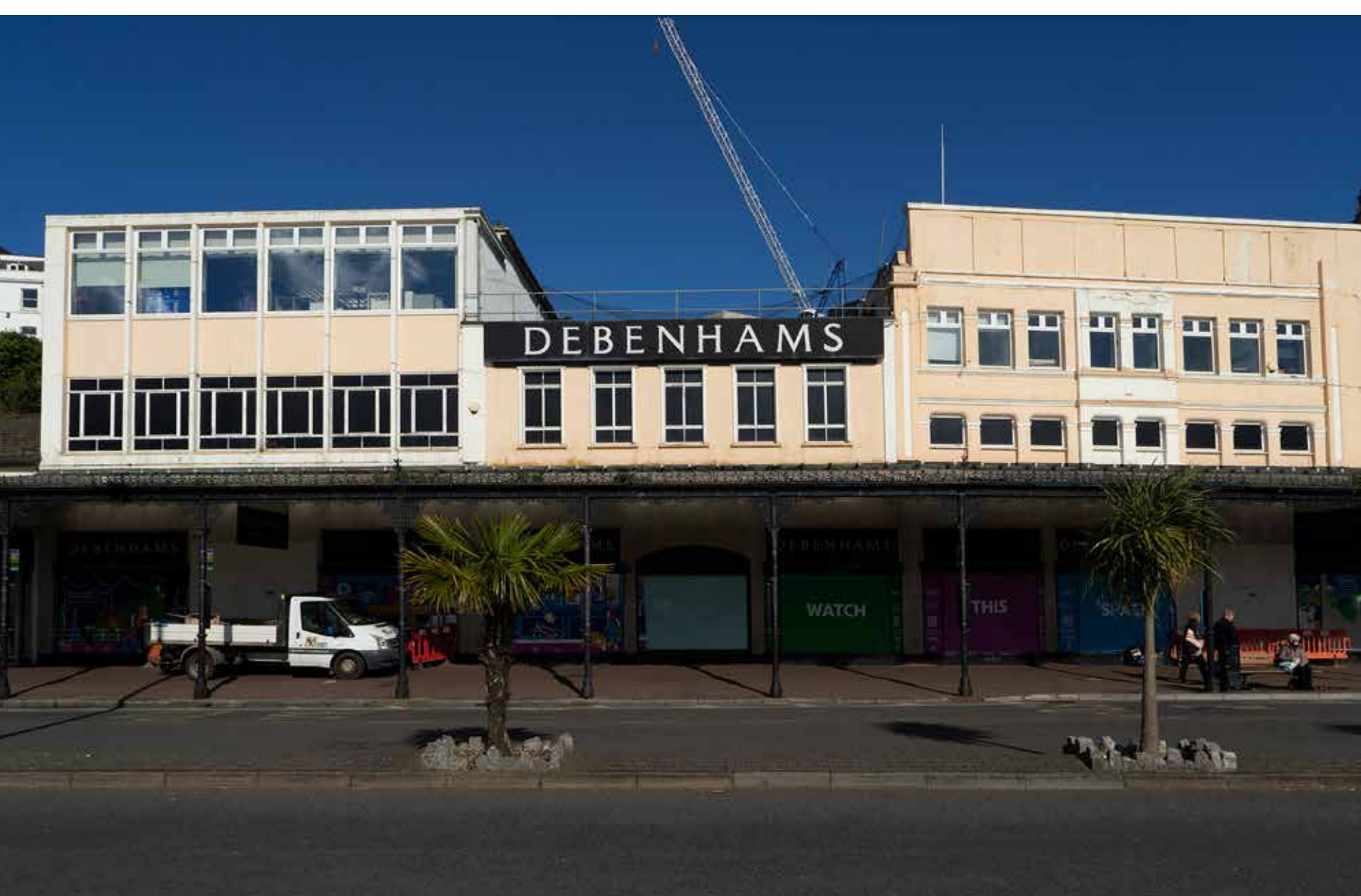
Above right: Photograph of flooding on The Strand in 2020. Image credit We Are South Devon Above: Debenhams current elevation. Image credit Sanders Studio
